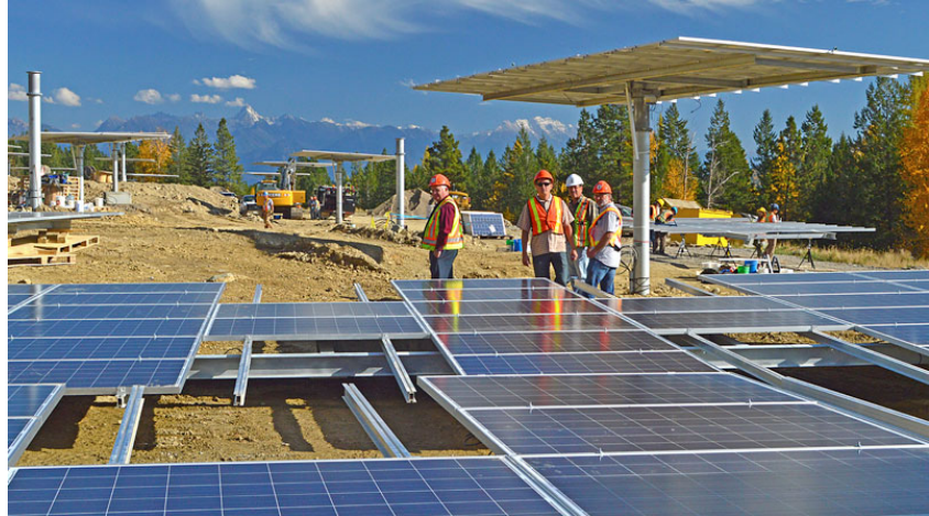
Construction of SunMine
