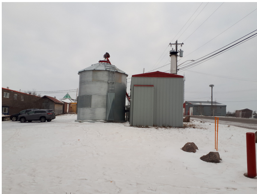
Figure 4. A wood pellet heating facility in Behchoko, N.W.T. November 12, 2019
